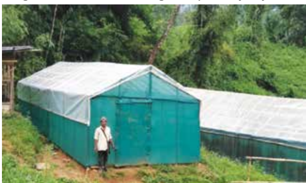
Fig 61. The two polyhouses constructed by the farmer
